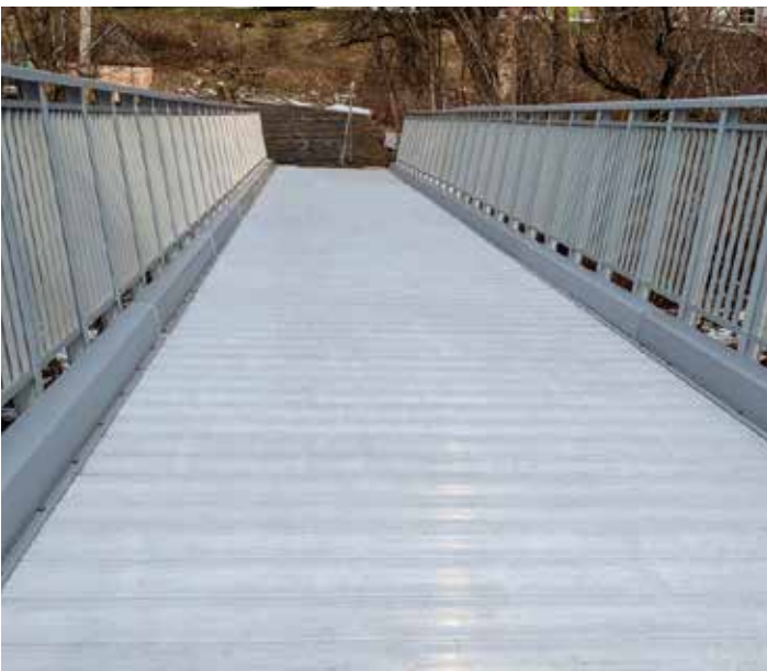
← Retrofit of existing bridge, Brome Lake, Quebec
