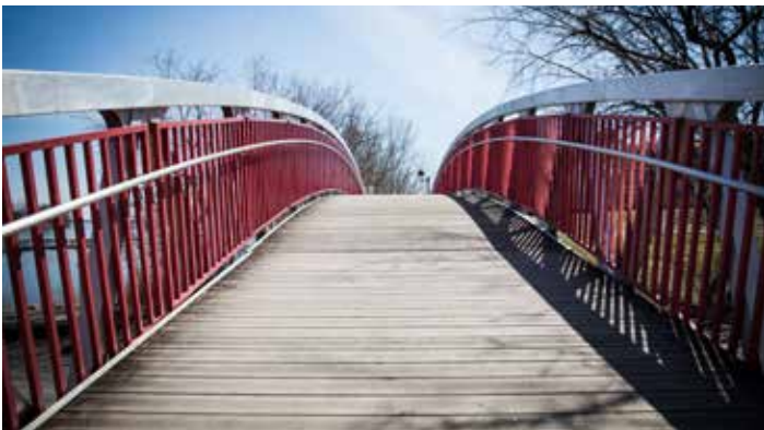
Figure 2. Condition 18 years later: no signs of wear (2020 photo)
