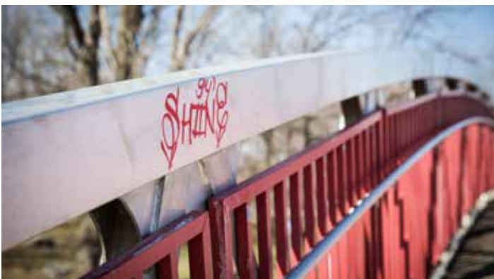
Figure 3. Unlike steel, aluminum can be easily sanded or pressure washed to remove graffiti without damaging the protective coating.
