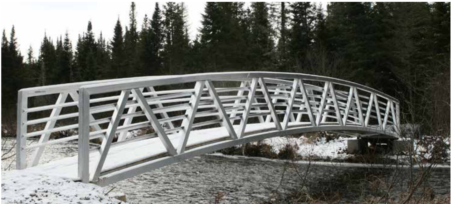
Figure 2. This aluminum bridge retains structural strength and corrosion resistance, even in extreme climate conditions.
