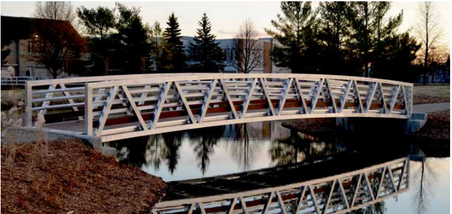
Figure 3. This aluminum bridge depicts a typical pedestrian aluminum bridge in an urban environment.
