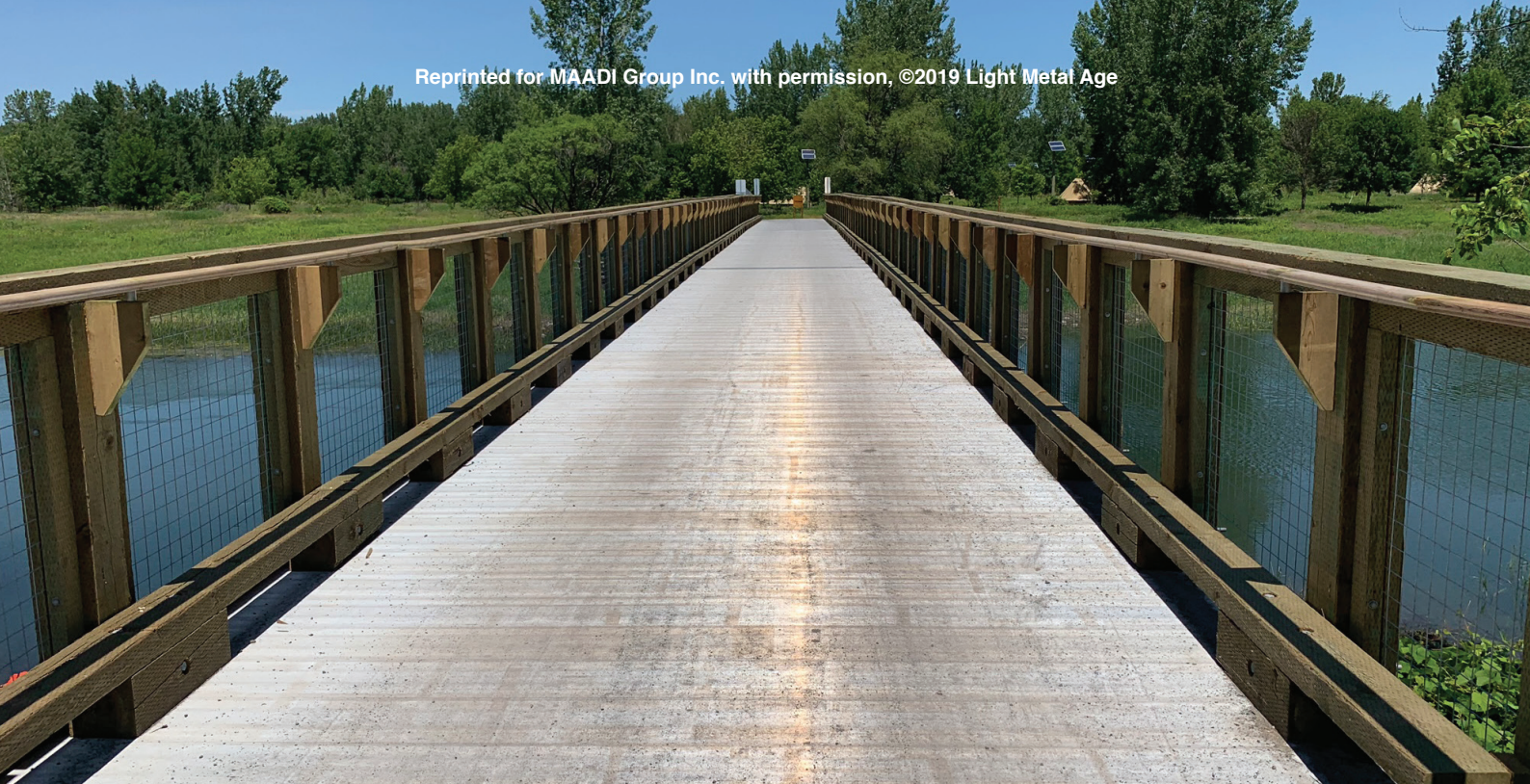
One of three GuarDeck bridges installed at the Parc national des Îles-de-Boucherville in Quebec, Canada, which spans 212 ft (64.5 m).
