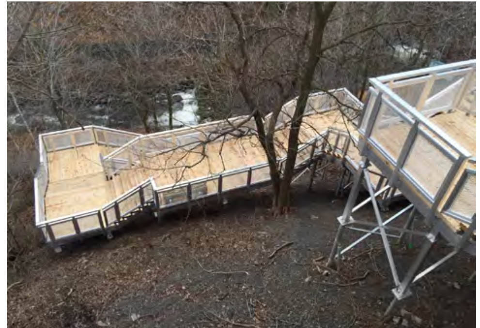
Fig 5.185 A safe low maintenance route through the trees of Parc de la Rivière-Beauport
