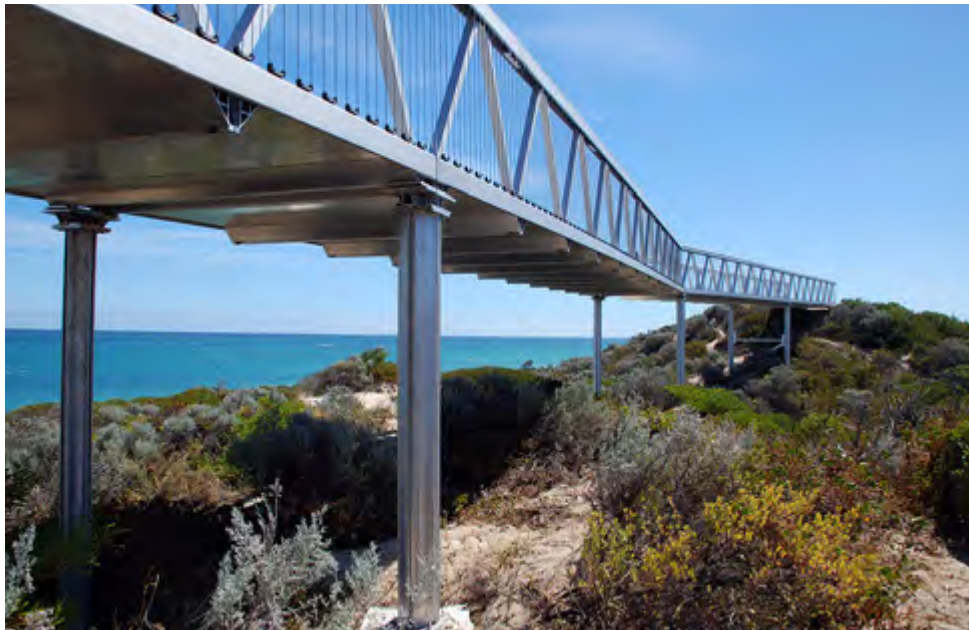
Fig 5.96 All aluminium Yanchep Bridge, designed and fabricated by Peter Maier Leichtbau
