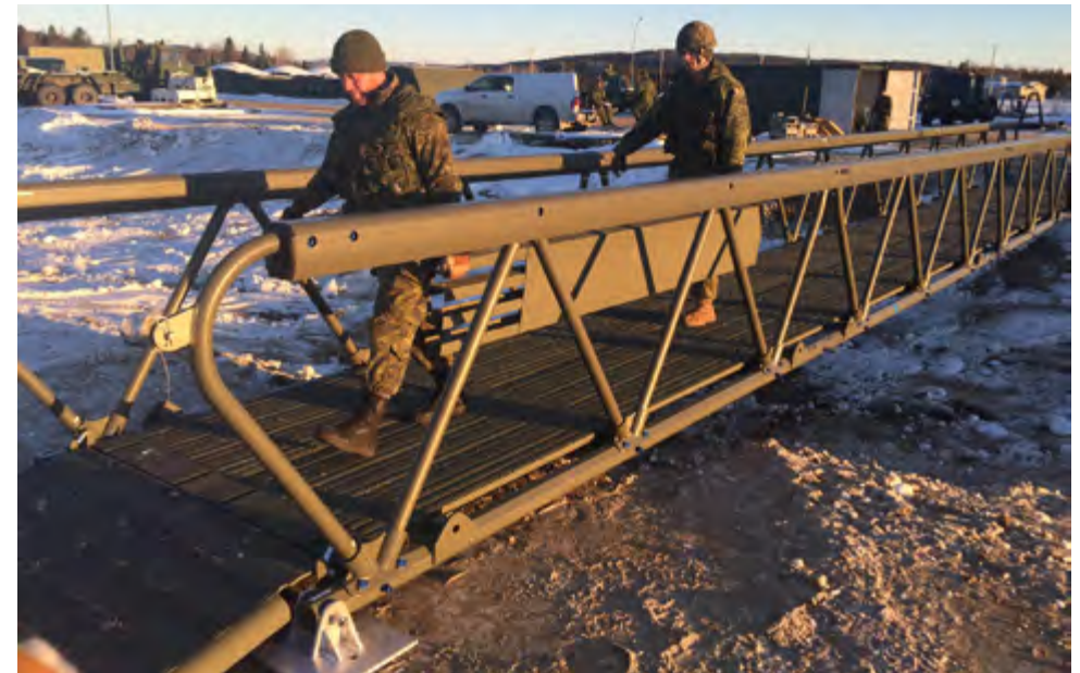
Fig 1.14 Deployable Military Bridge, Canada, designed and fabricated by MAADI Group, 2016
