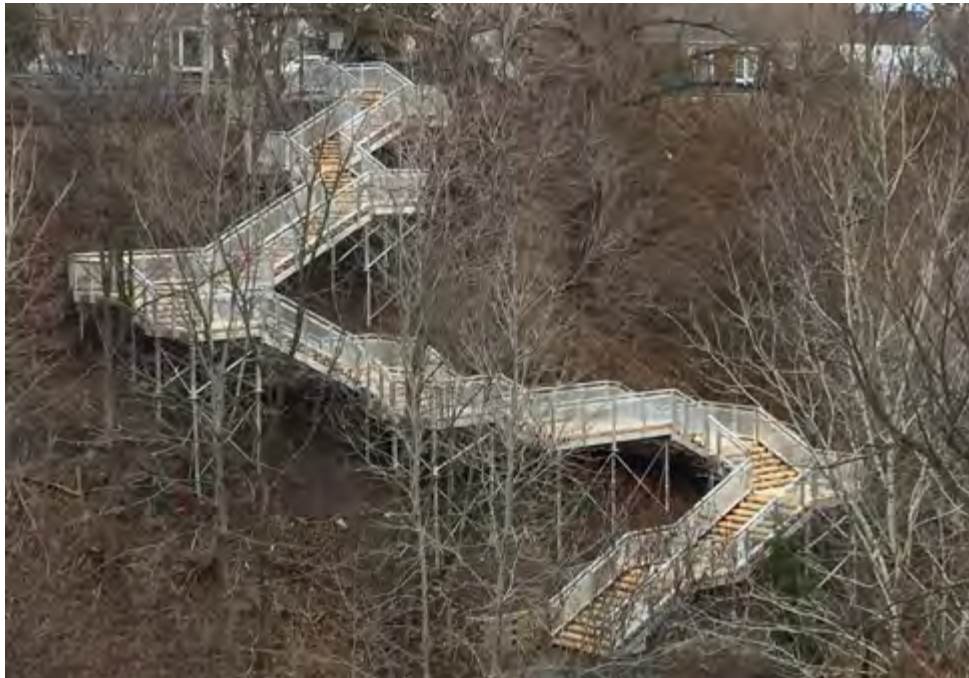
Fig 5.183 Aluminium Staircase descending 15m into Parc de la Rivière-Beauport
