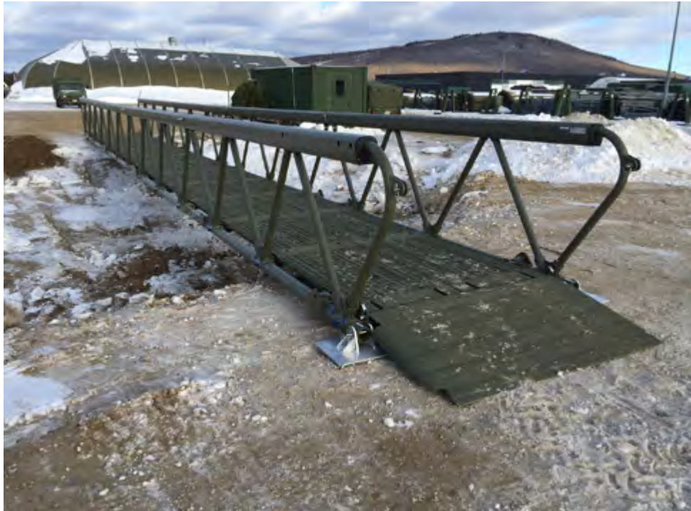
Fig 5.101 A prototype of a rapidly deployable military bridge with a maximum span of 16m
