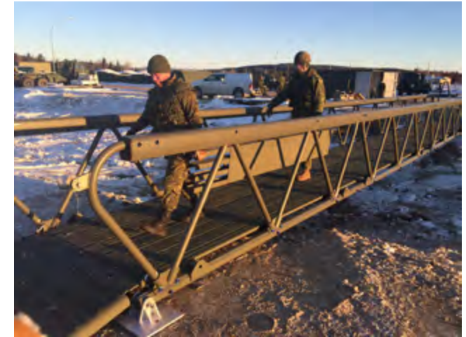
Fig 5.105 Military personnel using a rapidly deployable military bridge
