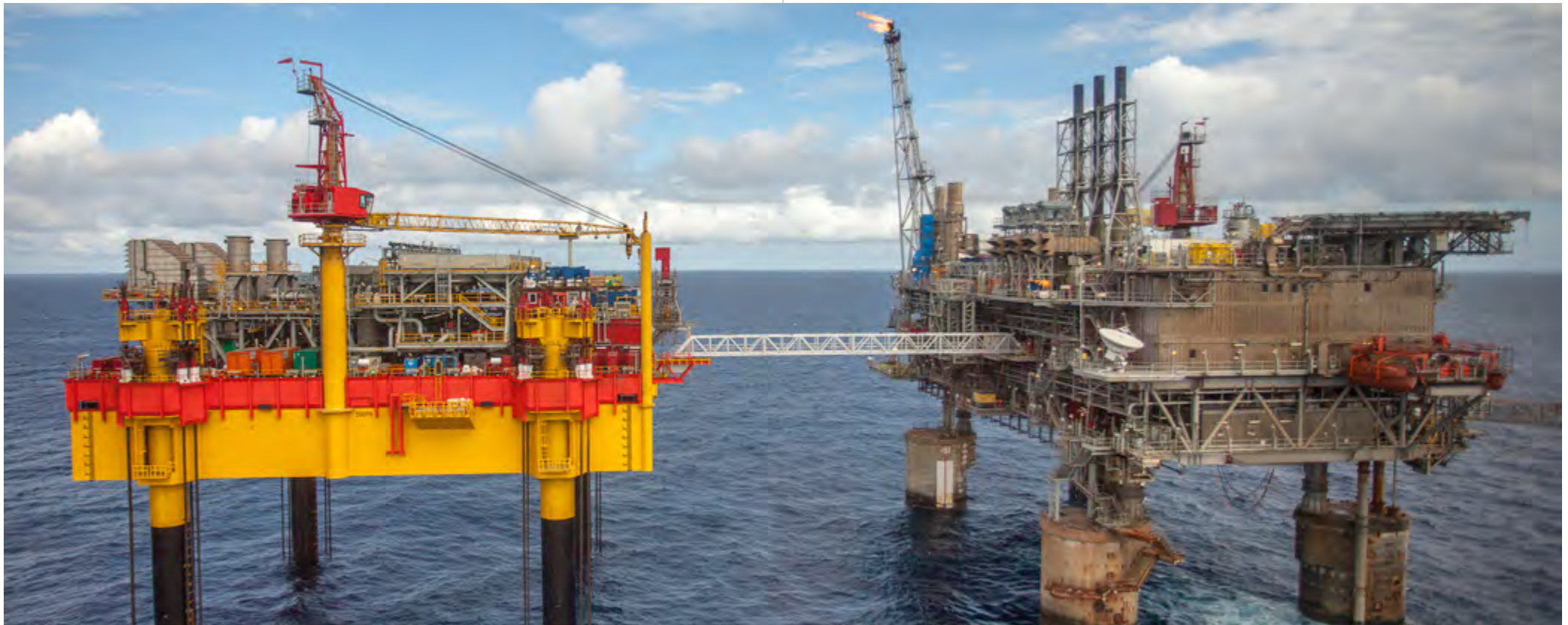
Fig 5.99 46.3m Oil Rig Pedestrian Bridge linking two offshore platforms, published with permission of the oil extraction company
