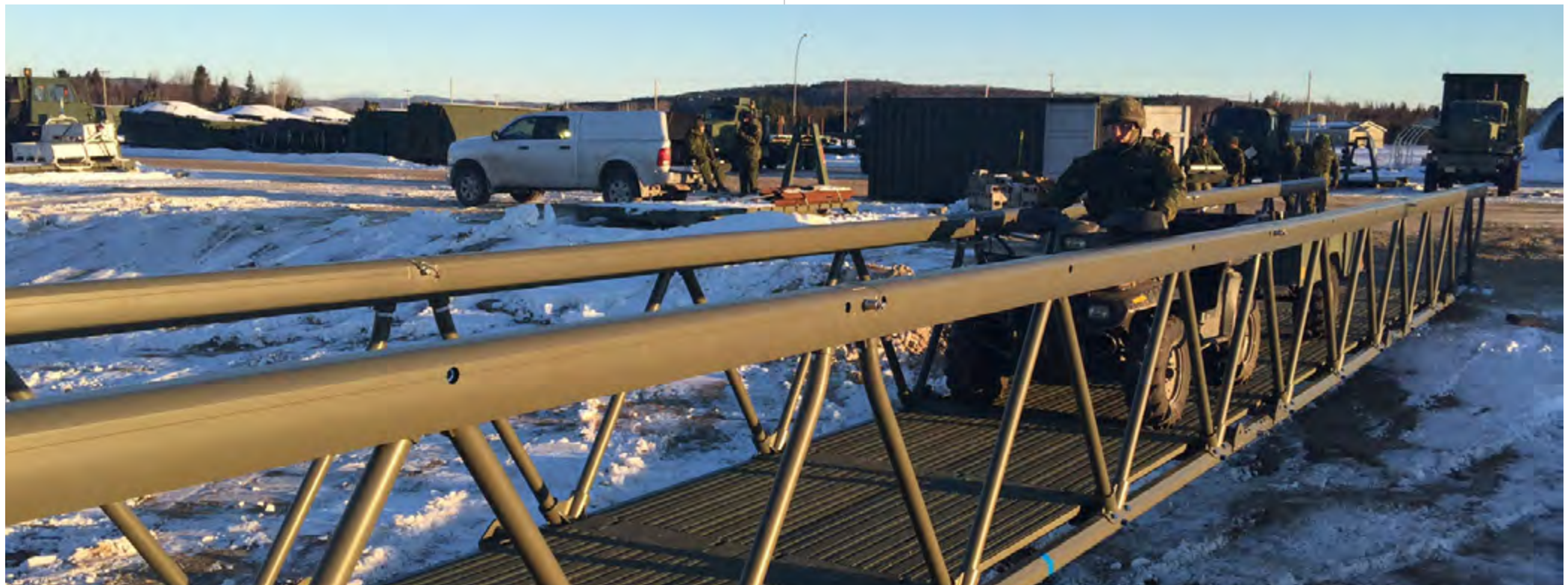
Fig 5.104 A rapidly deployable bridge can carry small vehicles, such as snowmobiles and quad bikes up to 500kg
