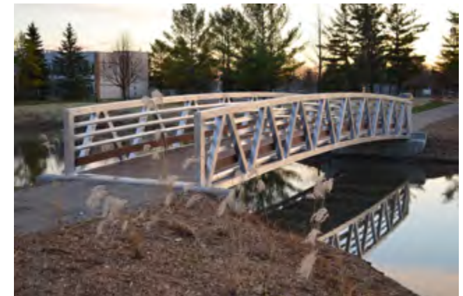
Fig 2.6 Welded aluminium pedestrian bridge by MAADI Group
