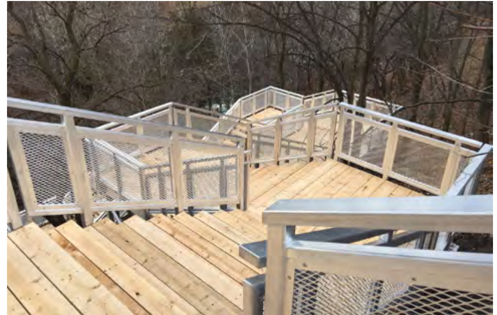
Fig 5.184 Timber treads and landing of the Aluminium Staircase in Parc de la Rivière-Beauport
