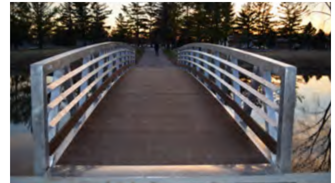
Fig 5.97 Equestrian Park Bridge, an aluminium bridge with a hardwood deck, designed and fabricated by MAADI Group
