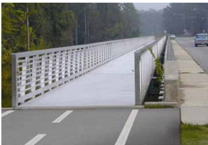
Figure 4. Cantilevered aluminum bike path (left) [C8], rapid bridge replacement in Ontario (right).
