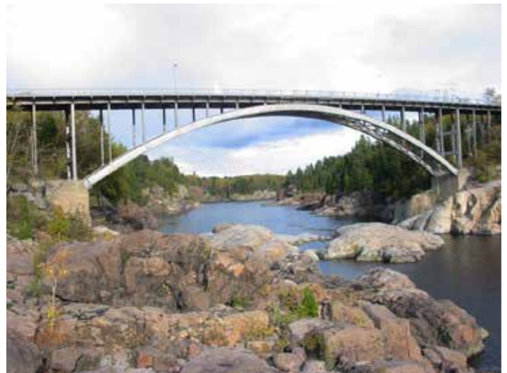
Figure 1. Arvida bridge in Saguenay, Quebec
