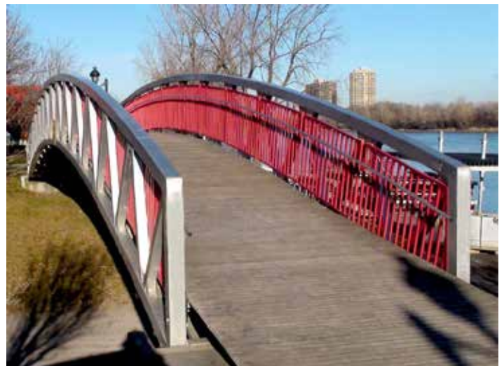
Figure 1. Aluminum pedestrian bridge installation
