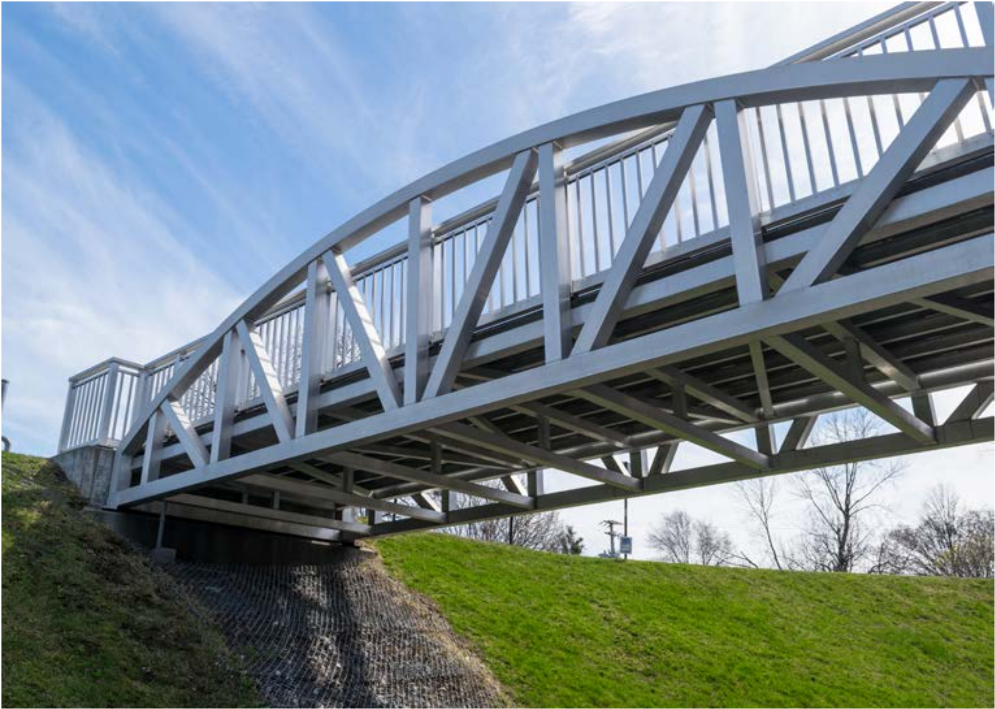
Design/build of a bowstring truss style bridge
