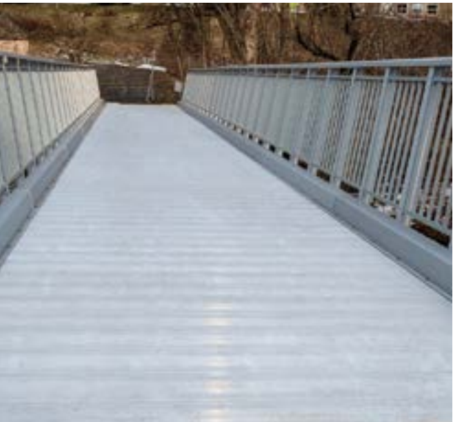
← Retrofit of existing bridge, Brome Lake, Quebec
