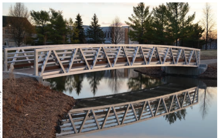
Equestrian Park Bridge, Blainville, Québec.
