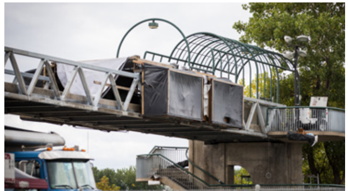
Figure 5. Condition 31 years later: repairs and maintenance work in 2014 and 2019 (2019 photo)
