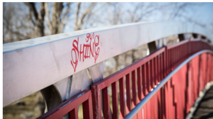
Figure 3. Unlike steel, aluminum can be easily sanded or pressure washed to remove graffiti without damaging the protective coating.
